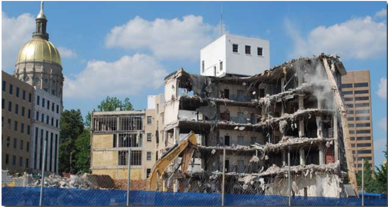
Demolition of the old Department of Transportation building
