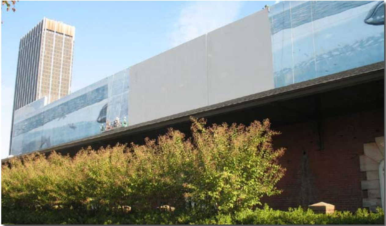
Renovation of the 90 Central Avenue Parking Deck
