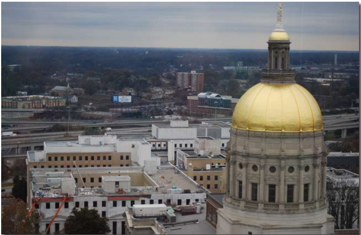
Capitol Hill Façade Repairs
